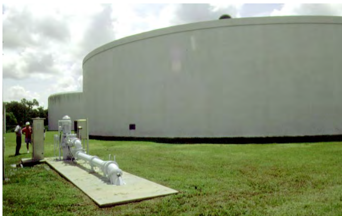
Figure 17. This ASR well in the foreground stores and recovers treated drinking water using the underlying aquifer at a depth of 100 to 130 m. The volume stored below ground during the low demand period and recovered in the high demand period at Cocoa, Florida, USA is ten times the volume of the two tanks behind. The unit storage cost of ASR was less than 2 per cent of the alternative cost of constructing additional tanks.
