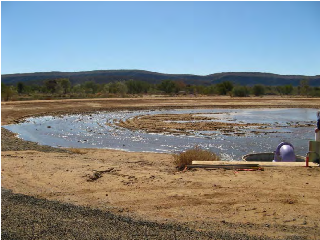
Figure 8. First fill of a soil aquifer treatment basin near Alice Springs ( photo courtesy Power Water Corp, NT )
