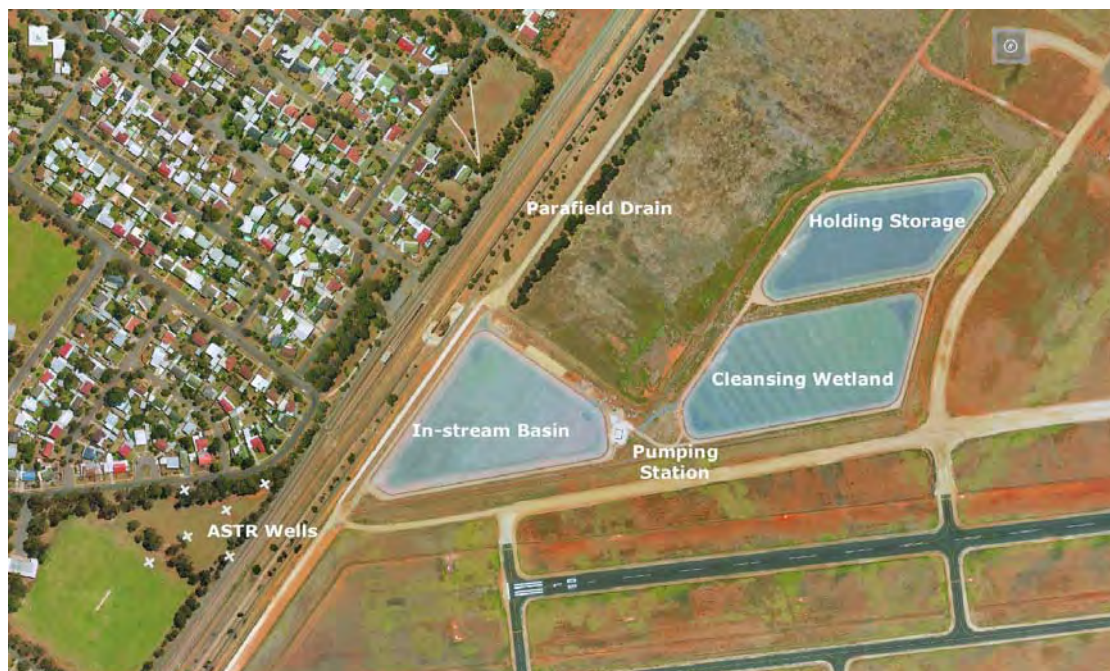
Figure 9 Salisbury ASTR stormwater to drinking water project. Shown are the drain, in-stream basin, holding storage and reedbed treatment (within Parafield airport). In lower left corner are the four outer injection wells and two inner recovery wells. In addition two ASR wells continue to operate on the northwestern side of the in-stream basin. (photograph courtesy of United Water)
